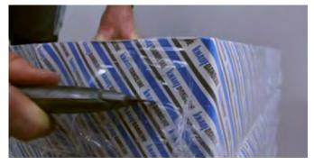
Cut the plastic wrapping by running a knife along the sides of the package. Do not cut the plactic on top of the package.
