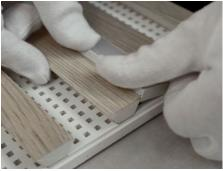
Push down to click the light strip into place and remove the protection film before installation.
