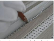
Point and mark the location for the cable and break the acoustic fleece on the backside through the perforation hole.
